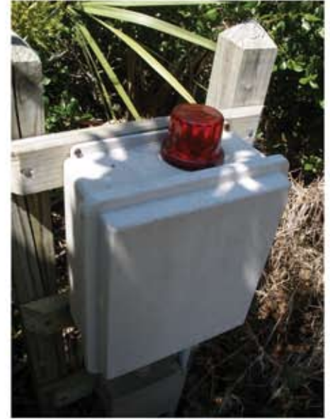
Figure 1: Alarm Control Panel Photo courtesy of Tom Robinson, Robinson Better Business Ideas
